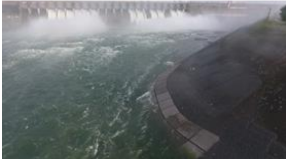
Fig. 13. Performance of divide bund after restoration [17]
