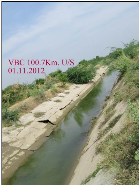
Photographs 4 and 5. Severe damage and pipings in the tail reach of Vadodara Branch Canal
