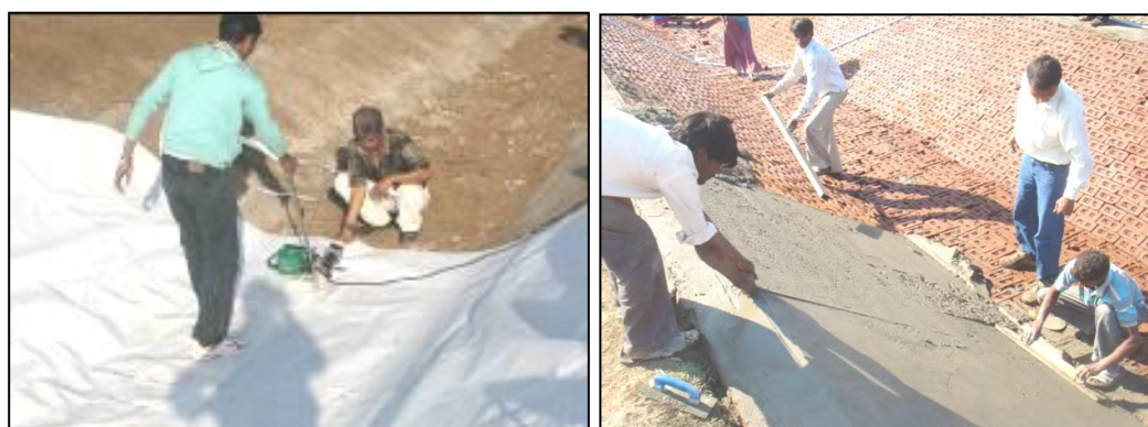
Photographs 6 and 7. Restoration of Tanchha Distributary
