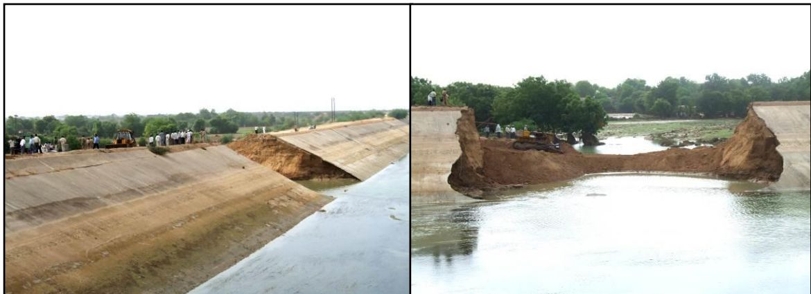
Photo – 5 and 6 Chiselled embankment
