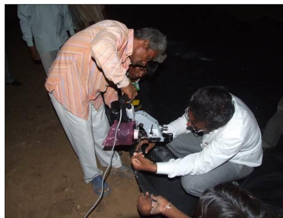
Photograph 8 and 9. Spreading, stitching and placing geotextile sheet
