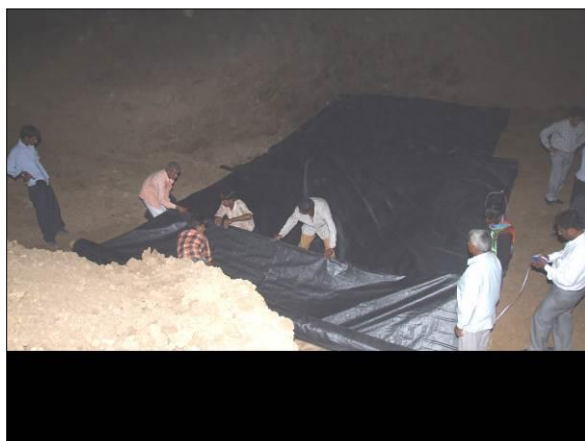
Photograph 8 and 9. Spreading, stitching and placing geotextile sheet
