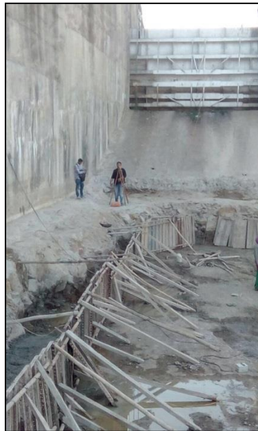
Fig. 4 Construction of Cut-off under Abutment
