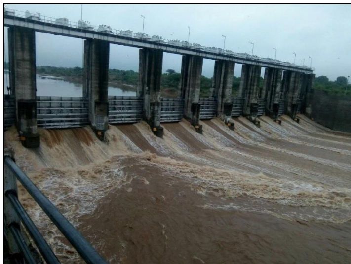
Fig. 6 Post-Repair Performance of Dam
