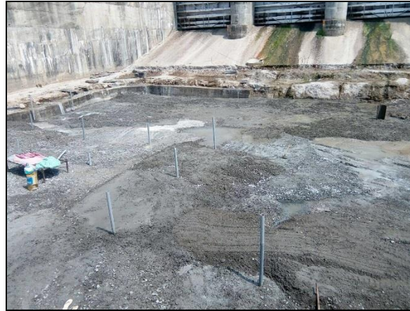
Fig. 5 Construction of Peripheral Cut-off
