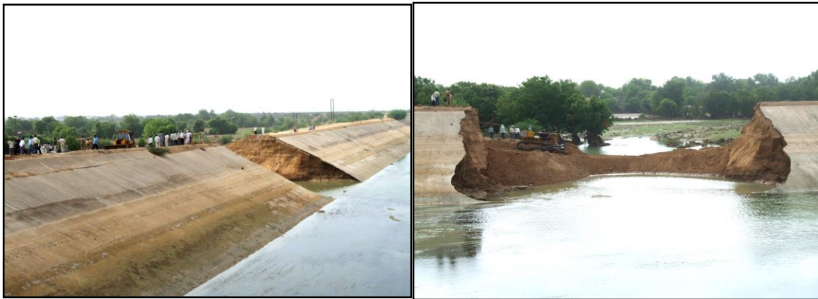
Photo – 5 and 6 Chiselled embankment
