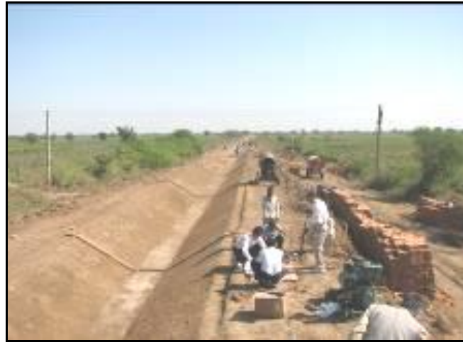
Photograph 15. Preparation of canal section
