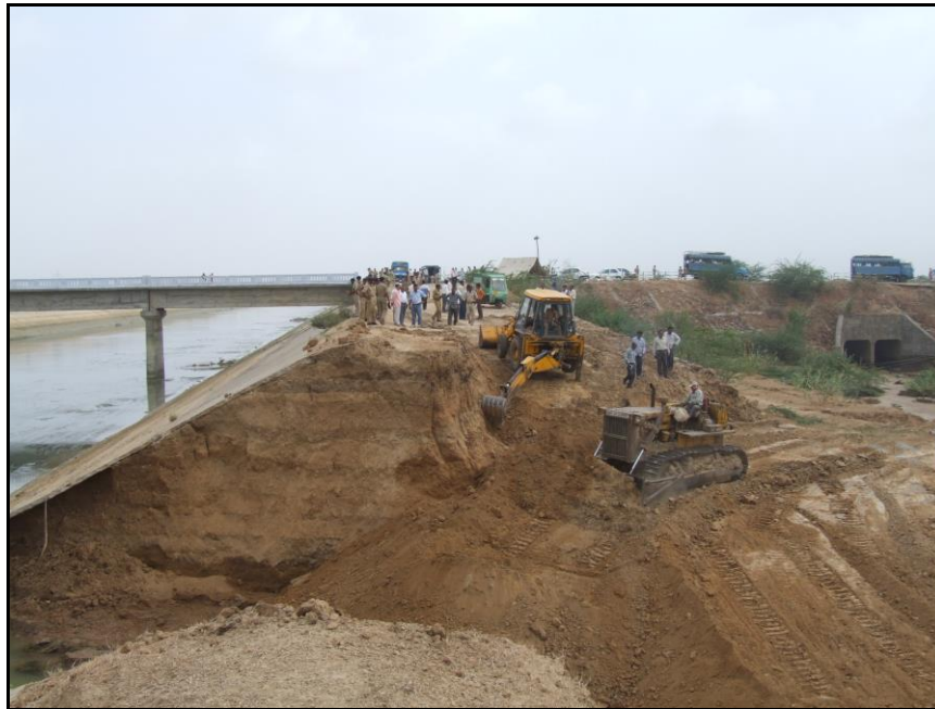
Photograph 7. Stratified strata of soil with no zoning or filters
