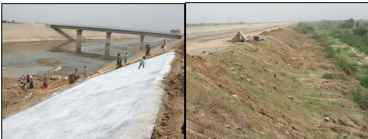
Photograph 10 and 11. Restored Main Canal embankment
