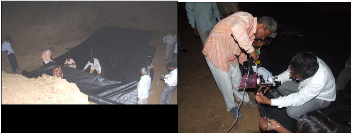
Photograph 8 and 9. Spreading, stitching and placing geosynthetic sheet
