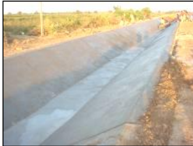
Photograph 17. Completed canal section
