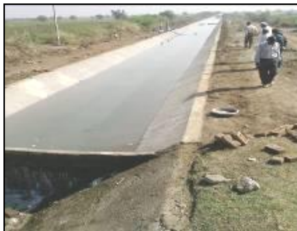
Photograph 18. Testing of completed canal section
