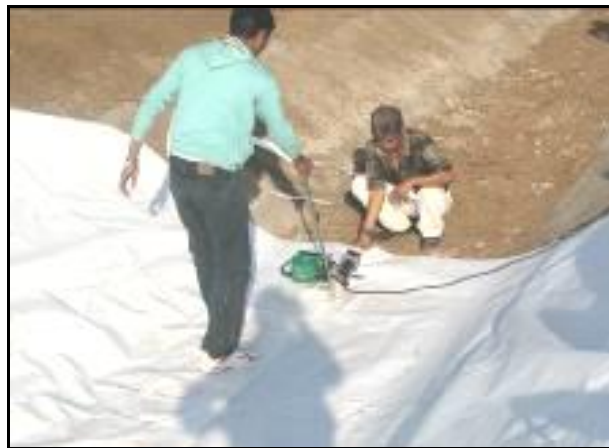
Photograph 16. Heat sealing of geomembrane
