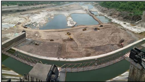
Figure 8. Execution of multistage secondary apron (Kapadia 2020)
