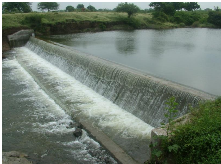
Figure 7. Checkdam across a medium sized river
