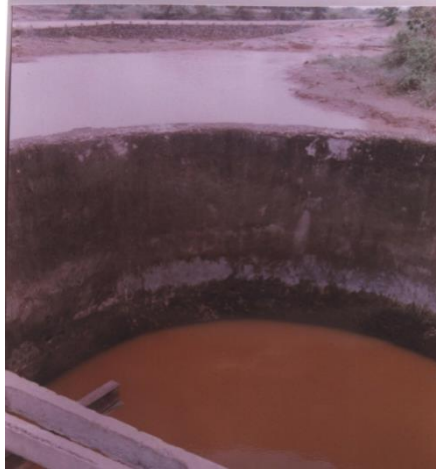
Figure 6. Well recharged in vicinity of checkdam
