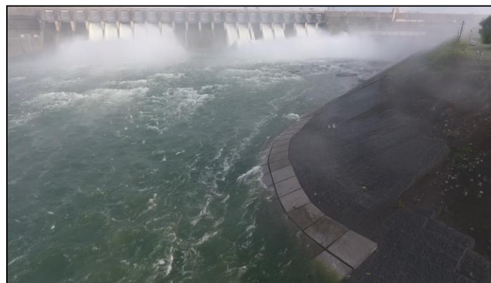
Figure 14. Actual performance of divide bund during monsoon of 2019
