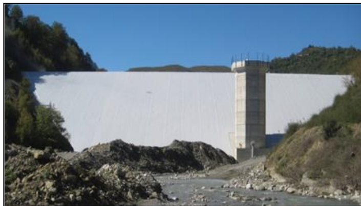
Figure 3. Murdari GFRD Dam Waterproofed with Wide, Pre-welded, Bands of Polymer 'Composite': PVC Geomembrane + PP geotextile
