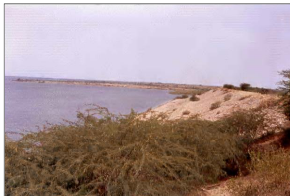
Figure 9. Kandaleru Dam, Tamilnadu, India
