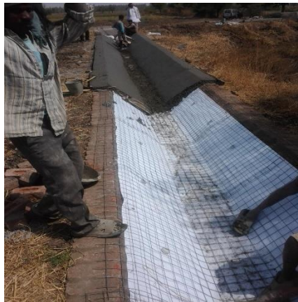
Figure 4. Canal lining with geomembrane
