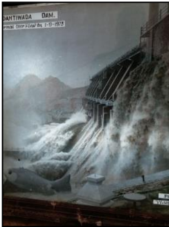
Figure 7. Dantiwada Dam – actual flood much more than the design flood
