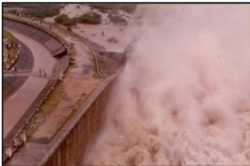
Figure 8. Dantiwada Dam – endangered due to heavy flood
